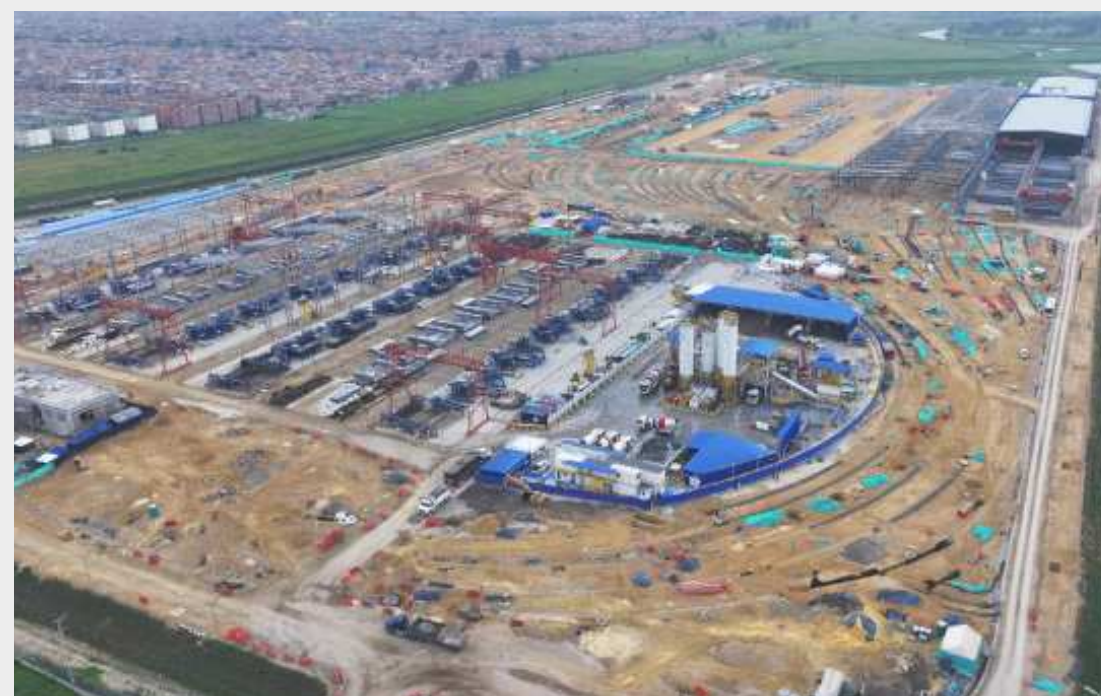
Avance General Patio Taller
